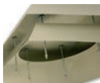
Hood with natural outlet air due to differential pressure
