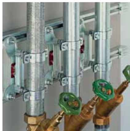
Vibration-decoupled water pipe anchor points
