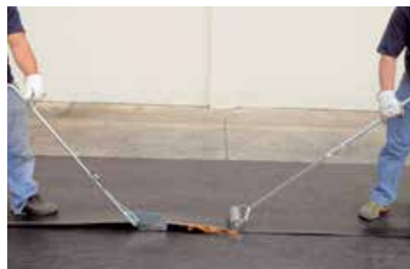
Combined use of Lap Torch and Seam Roller
